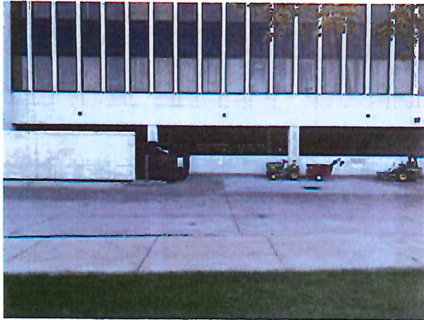
A. Fence and Gate Infill Area
