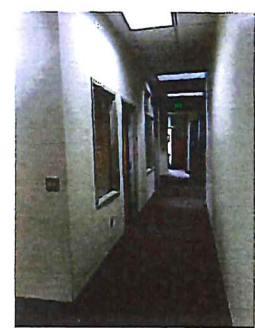
PHOTO 5 - CORRIDOR LOCATION OF NEW DOOR
