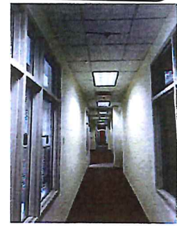
PHOTO 6 - CORRIDOR LOCATION OF NEW DOOR
