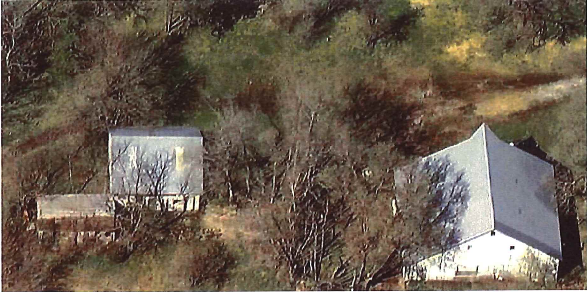
Barn & outbuildings from south
