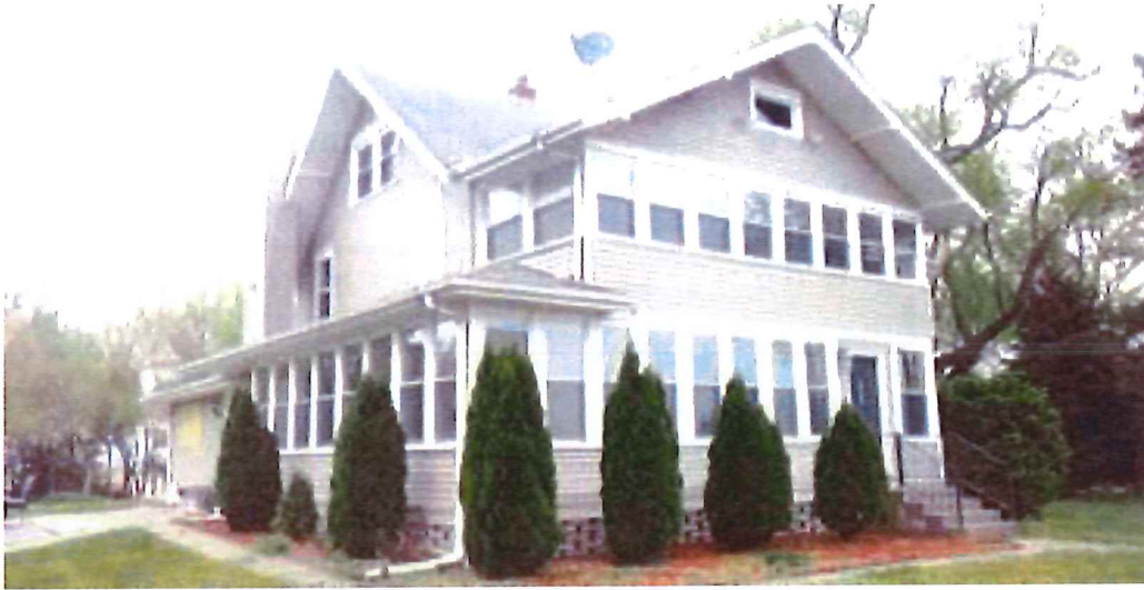
South (left) and east (right) facades of farmhouse
