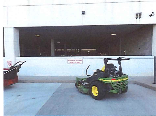
B. Cut Egress Opening in Wall
