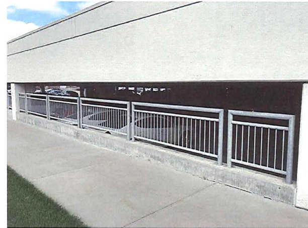
D. County-City Parking Deck
