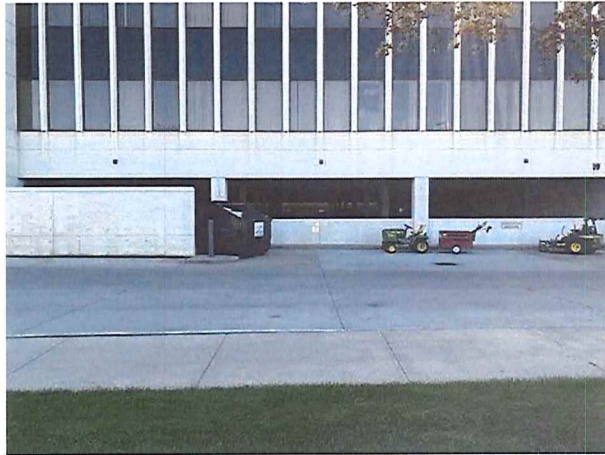
A. Fence and Gate Infill Area
