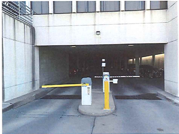
C. Remove Control Arms & Add Rolling Steel Garage Doors
