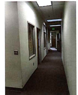
PHOTO 5 - CORRIDOR LOCATION OF NEW DOOR
