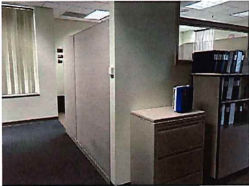
PHOTO 3 - LOCATION FOR NEW WALLS AND DOOR FRAMES
