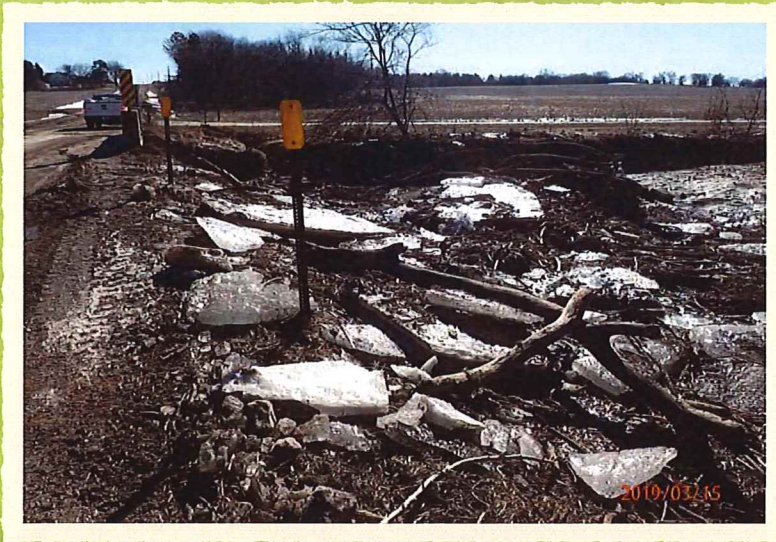
Bridge B-133 located on Agnew East of North 56
