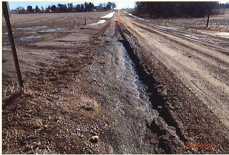
Agnew Road east of Hwy 77
