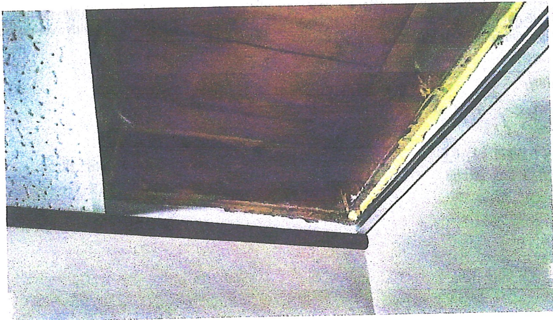
1B. Roof Decking Below SE Corner – Living Room.
