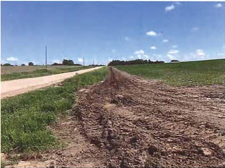
Photo No. 6 Looking north along South 82 nd Street from near Bennet Road showing permanent easement area Taken by Steve Medill June 7, 2019
