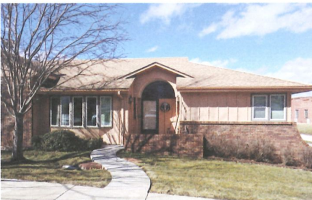
This Auburn property is one of the four homes purchased by the foundation this year.
