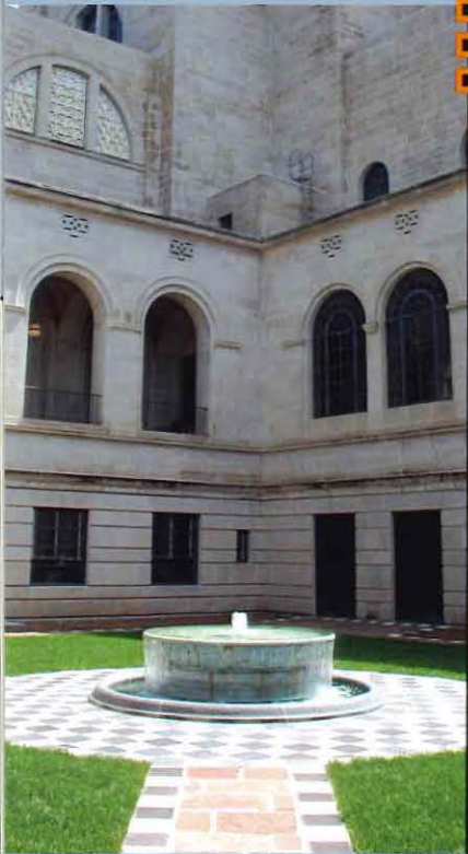
Today, the fountains are in place, awaiting the landscape restoration of the courtyards to make the builder's vision complete.
