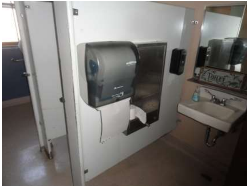
SUBJECT PHOTOGRAPH: SHOWING TYPICAL RESTROOM FINISH.
