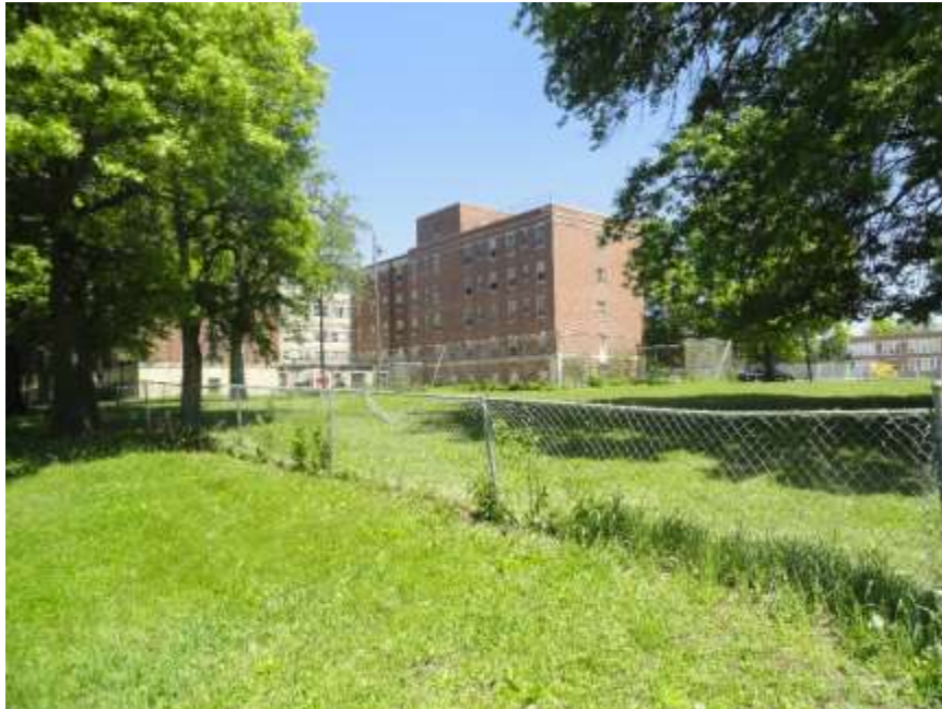
SITE PHOTOGRAPH: LOOKING NORTHEAST ACROSS SUBJECT SITE FROM NEAR THE SOUTHWEST CORNER OF SUBJECT SITE.
