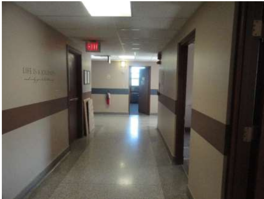
SUBJECT PHOTOGRAPH: SHOWING TYPICAL HALLWAY FINISH. SHOWING COMMON AREA.
