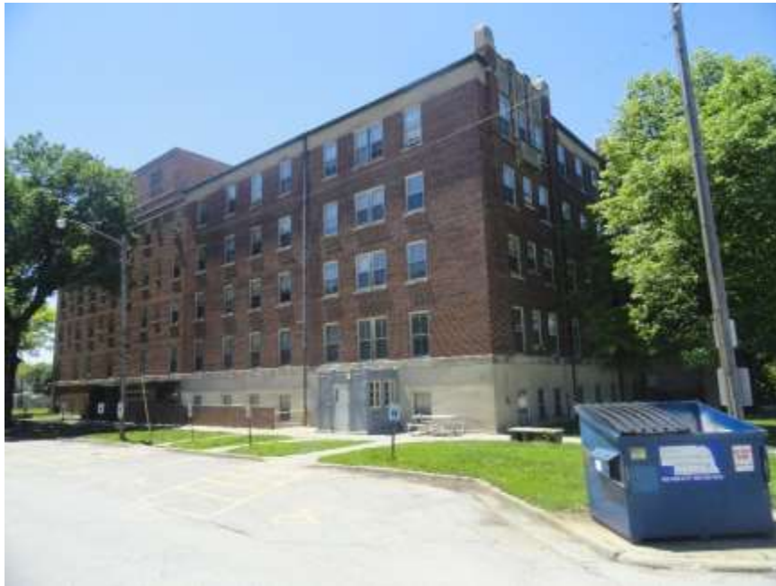
SUBJECT PHOTOGRAPH: LOOKING SOUTHWEST AT EAST EXTERIOR ELEVATION OF SUBJECT IMPROVEMENT.
