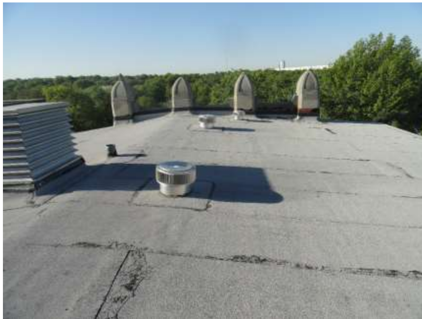
SUBJECT PHOTOGRAPH: SHOWING ROOF FINISH.
