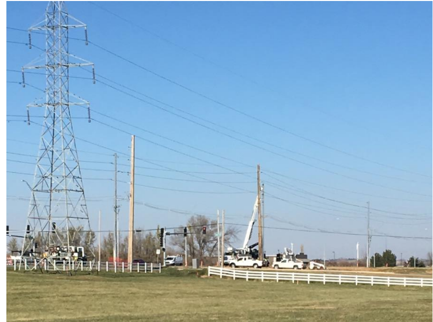
Since October: Utility pre-work Photo as of today, Nov. 15, 2018
