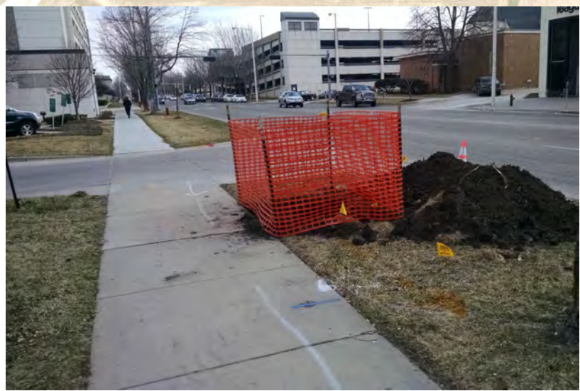
ORANGE PLASTIC CONSTRUCTION FENCE EXAMPLE
