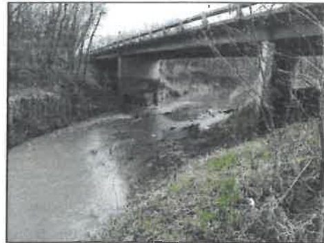
Figure 7-12: Old Cheney Rd Bridge Piers Exposed
