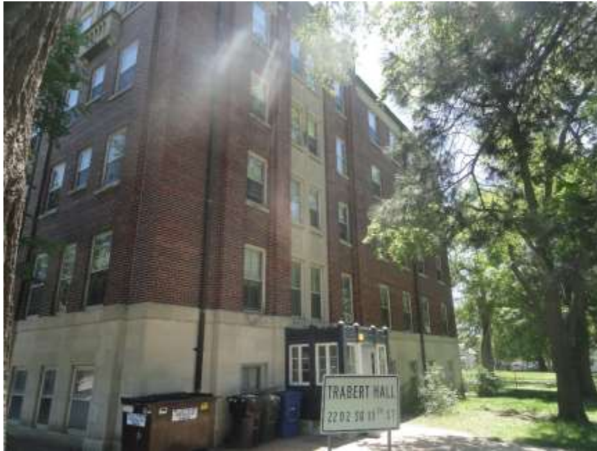
SUBJECT PHOTOGRAPH: LOOKING SOUTHEAST AT WEST EXTERIOR ELEVATION OF SUBJECT IMPROVEMENT.
