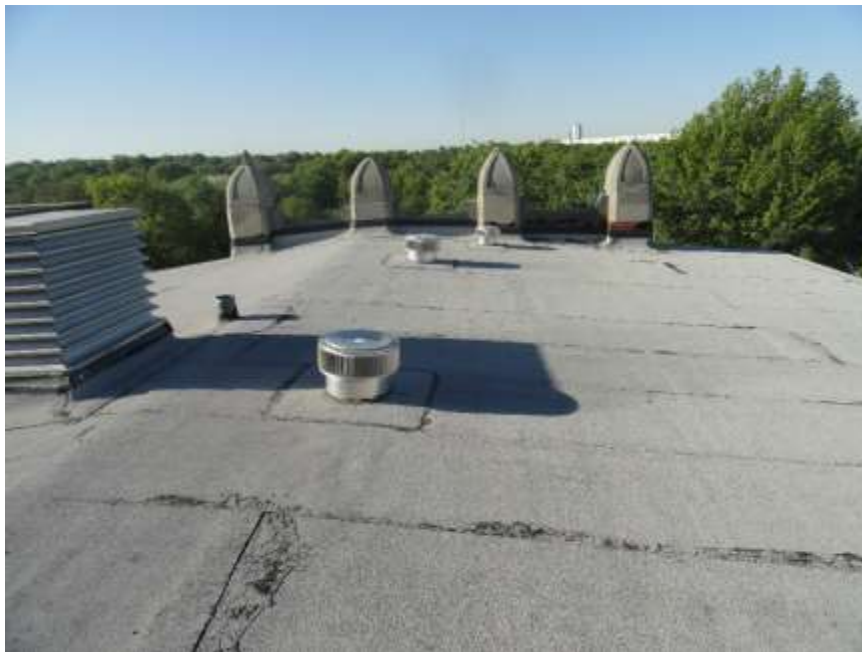
SUBJECT PHOTOGRAPH: SHOWING ROOF FINISH.
