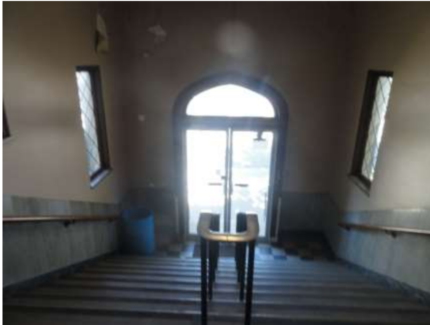
SUBJECT PHOTOGRAPH: SHOWING MAIN ENTRANCE / VESTIBULE AREA.
