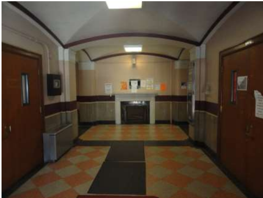
SUBJECT PHOTOGRAPH: SHOWING MAIN ENTRANCE / VESTIBULE AREA.
