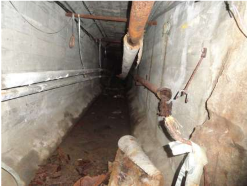
SUBJECT PHOTOGRAPH: SHOWING TUNNEL AREA ACCESSED VIA LOWER LEVEL.
