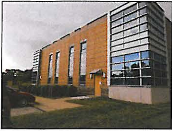
Brick and window envelope
