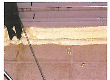
Weatherization Sealing of Air Gap Between Wall and Roof Deck
