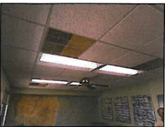
Airport Terminal T8 Lighting
