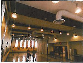
Carnegie Building Lighting
