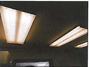
Existing Solid Waste T8 Lighting
