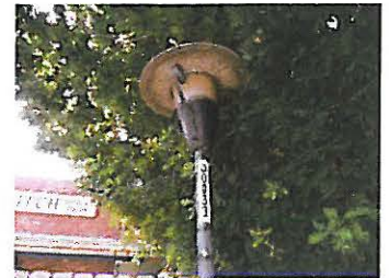
Aged and Distressed Pole To Be Replaced
