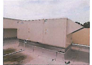
Typical VAV Rooftop Unit
