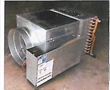
New VAV terminal
