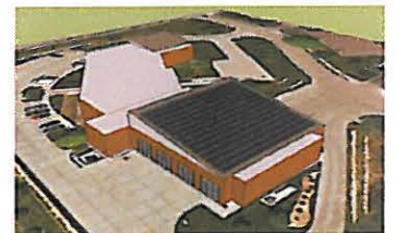
Computer Rendering of a 100kW PV Array on the roof of Fire Station #5.
