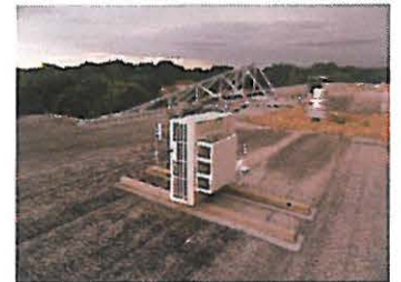
Substantial De-Mineralization on Community Health Building Roof
