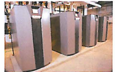
Modern Condensing Boiler With Higher turndown
