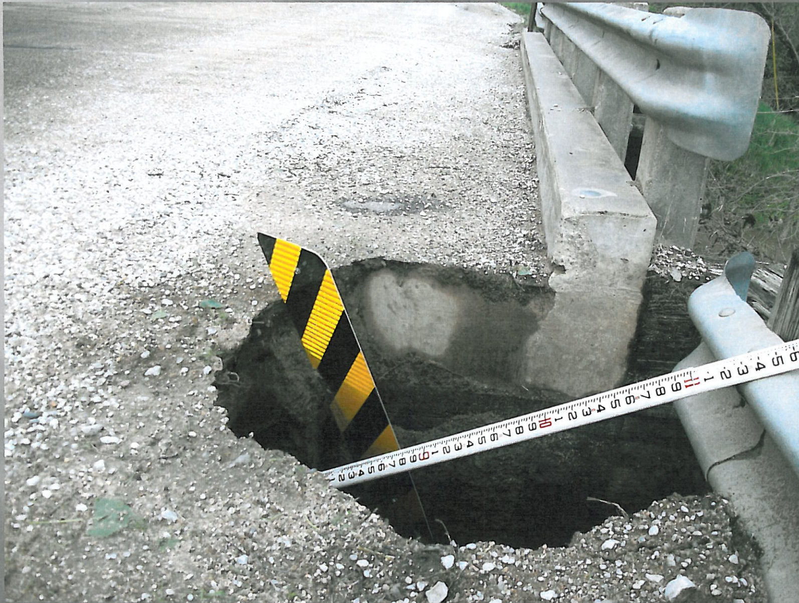
Bridge N-19 had a 10 foot scour hole behind the abutment.
