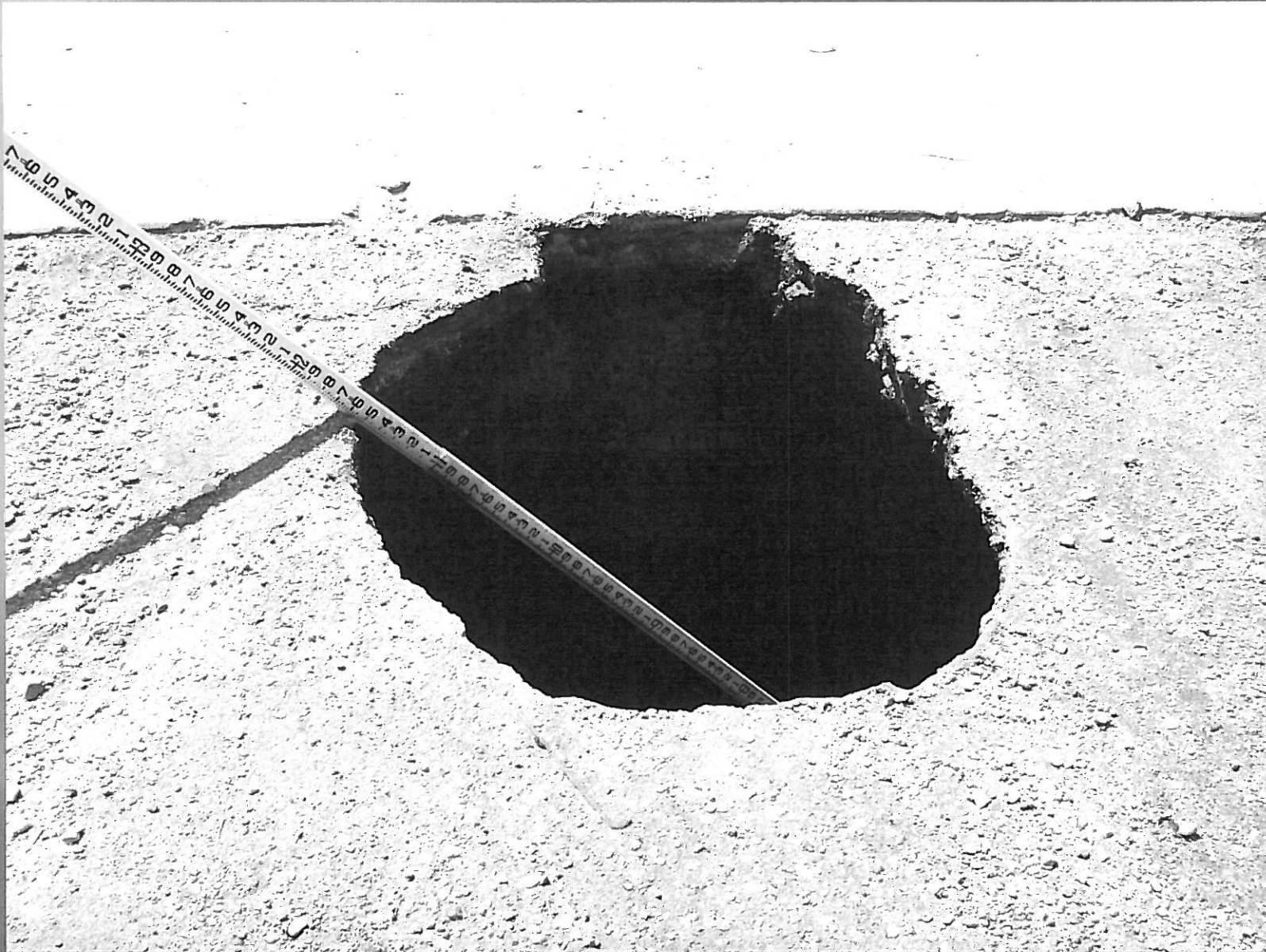
Bridge T-171 had a 11 foot scour hole behind the abutment.
