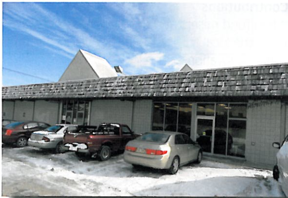
Region V Services purchased a building at 3151 South Street for L3 to use for their Plaza Connection Day Service program.
