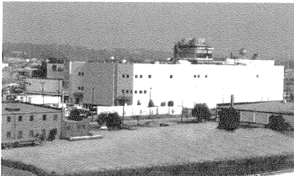
ENERGY SYSTEMS COMPANY CALIFORNIA STREET THERMAL ENERGY PLANT NEW CONSTRUCTION OMAHA, NEBRASKA • 22,000 Tons Chilled Water Capacity • 160,000 lbs/hour Steam Capacity • 7,196 LF Steam/Chilled Water Utility Extension
