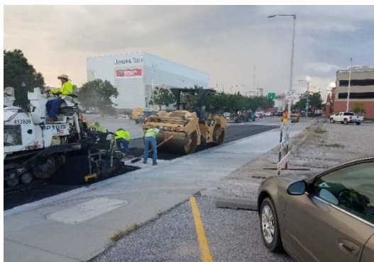
Mill and overlay project
