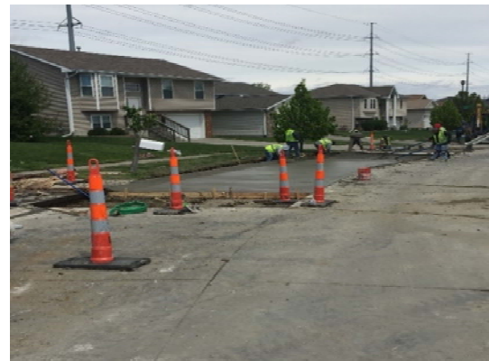
Pavement repair project
