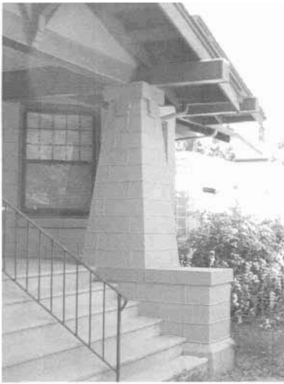
Detail of west porch pier, 2009, showing raised joints.
