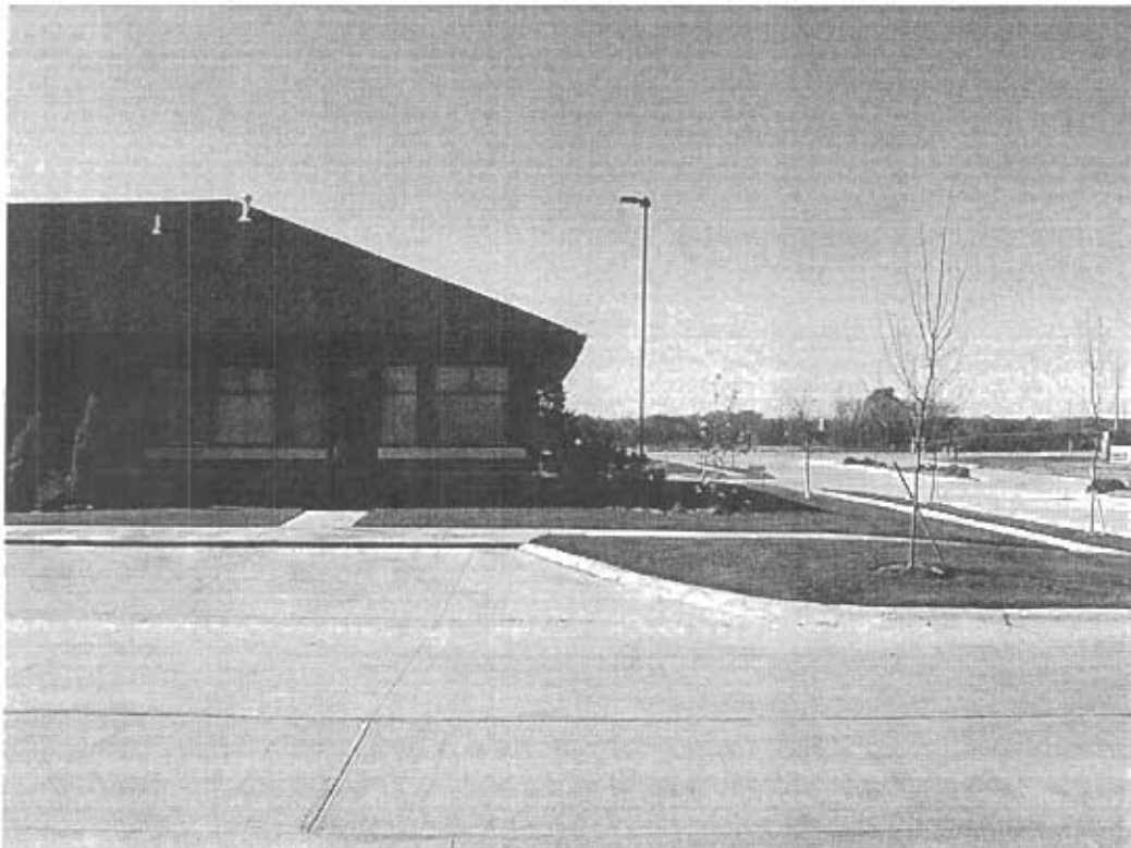
Good sidewalk connection into commercial pad site
