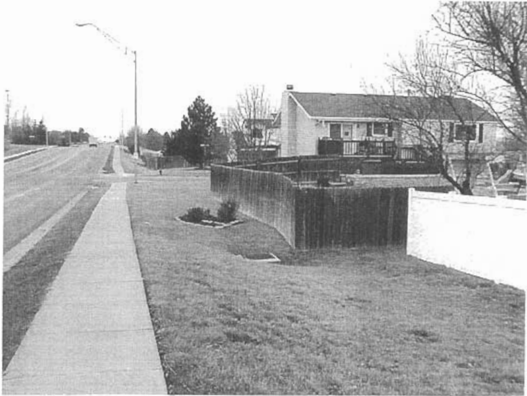
An arterial with the sidewalk too close to curb
