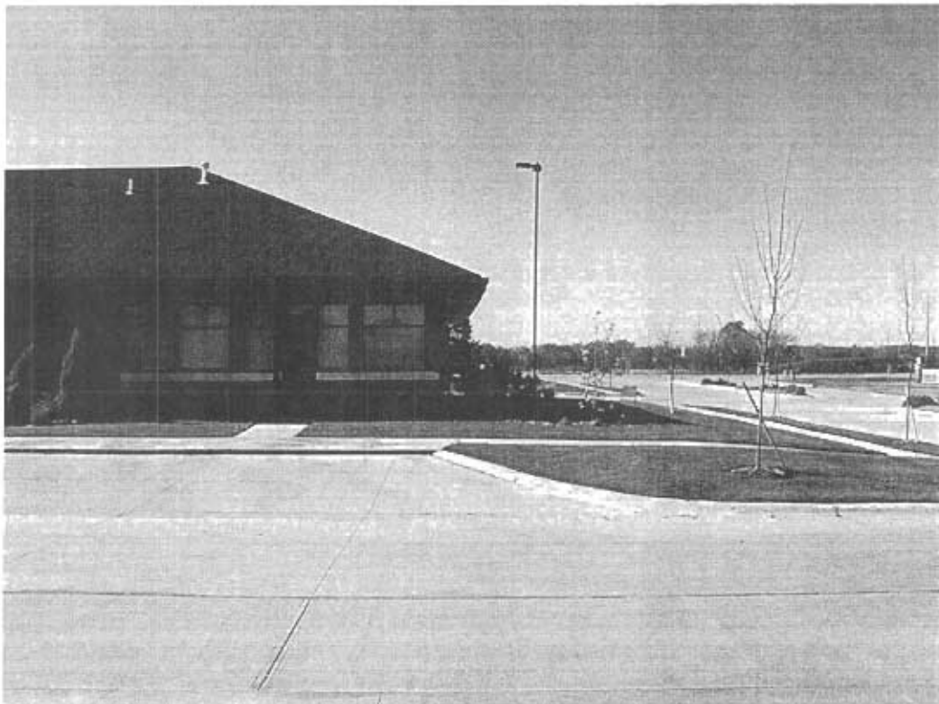
Good sidewalk connection into commercial pad site
